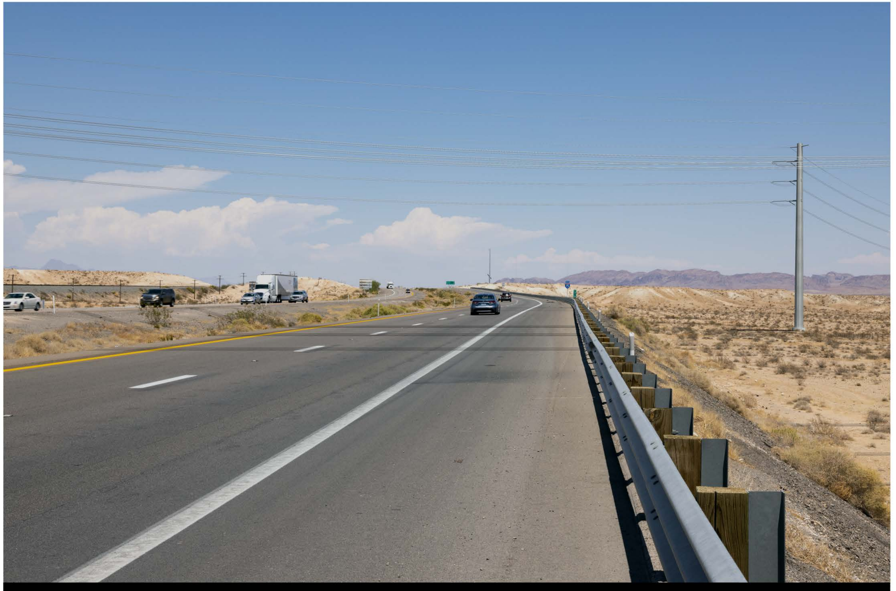
Figure 6b CHUCKWALLA SOLAR PROJECT NORTHBOUND I-15 LOOKING NORTHEAST - SIMULATION
