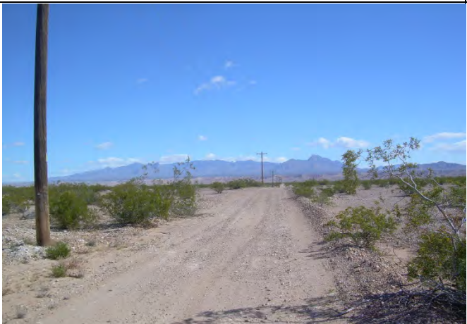
View of transmission line located on the southern portion of the Subject Property.
