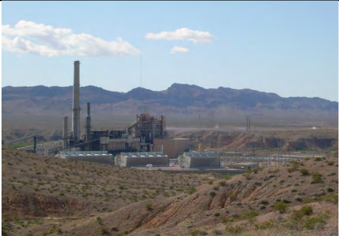
View of Reid Gardner Generation facility further south of the Subject Property.
