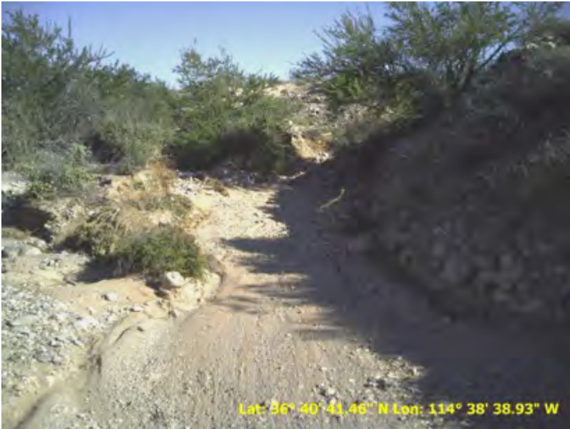
Photo 4. M02. Potentially jurisdictional lower reach of this drainage, showing presence of bed and bank, sediment sorting and deposition, and destruction of terrestrial vegetation.
