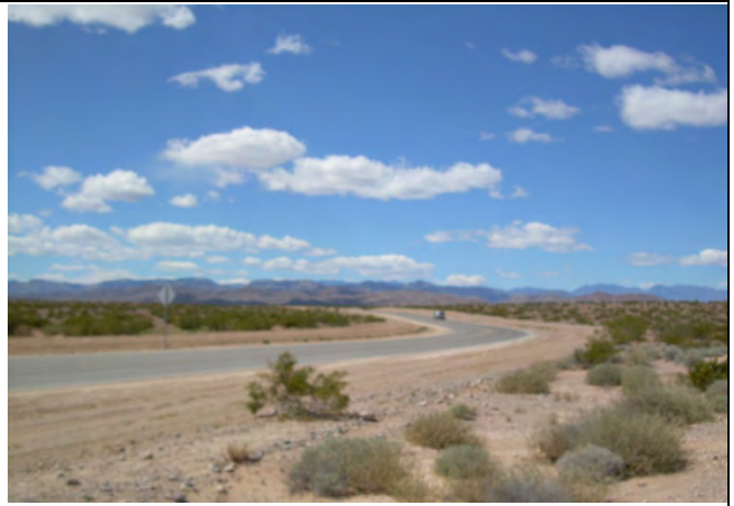
View of Lytle Lane located on the northwest portion of the Subject Property facing west.
