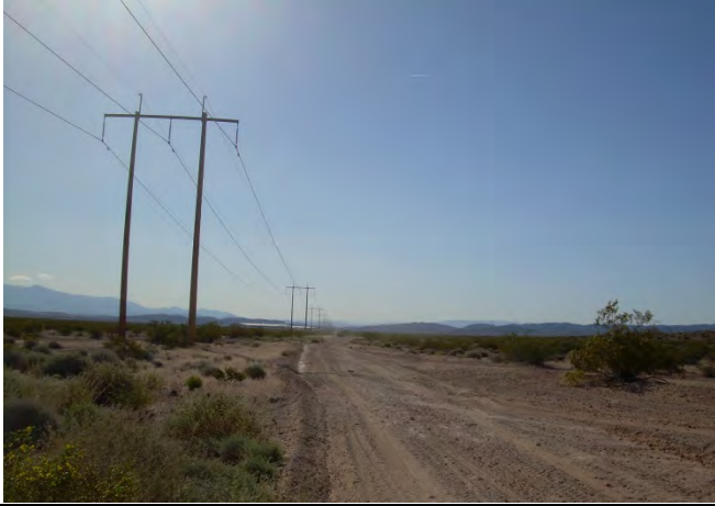
View of the northern Subject Property boundary facing southeast along the northern transmission line.
