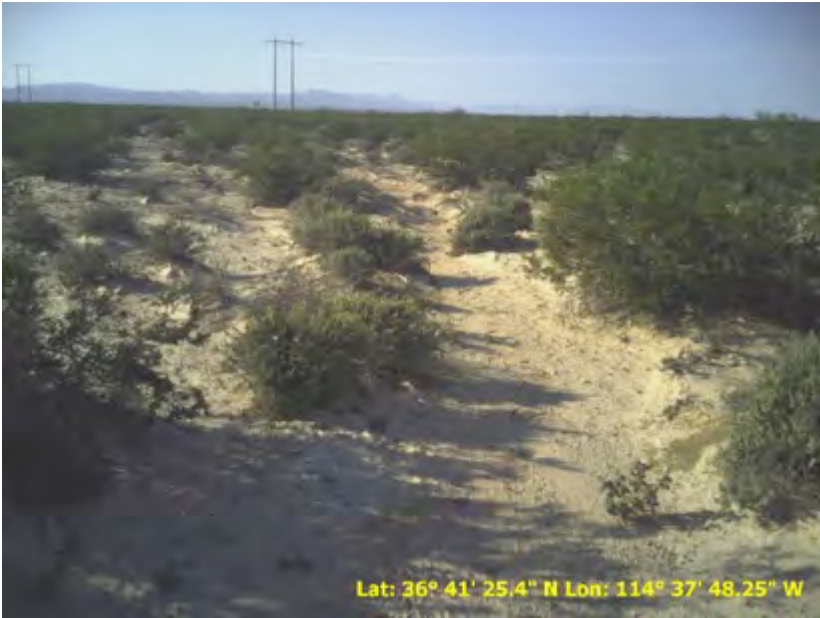
Photo 13. M06. A swale on the east boundary of the project site showing movement of fine sediment during the recent precipitation event. Note no change in vegetation from surrounding uplands.
