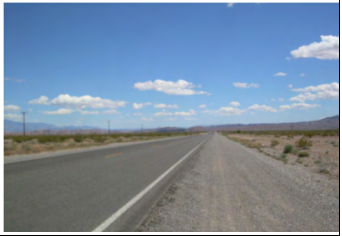
View of Highway 168 that runs through the Subject Property.
