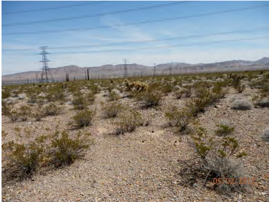
Representative habitat near Harry Allen substation (May 2012)
