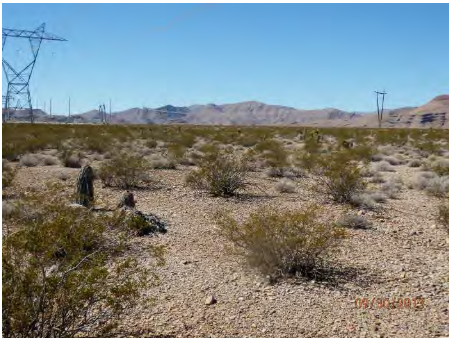
Representative habitat on the 230 kV re-route ROW (Oct 2013)
